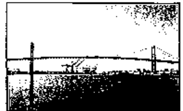
Vincent Thomas Bridge
